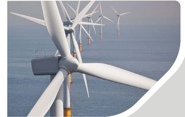
Race Bank offshore wind farm
